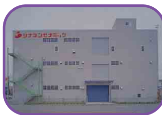
The completion of this new production facility will enable sinanen to triple output of Zeomic.
