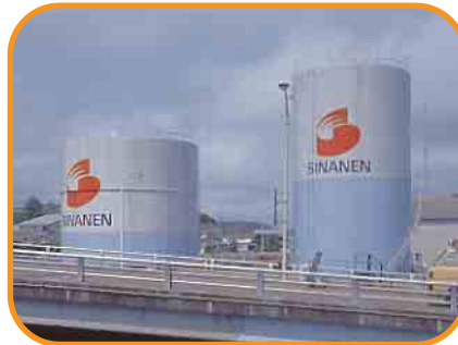
Sinanen's oil storage facilities play a key role in ensuring the safe and efficient distribution of oil products throughout Japan
