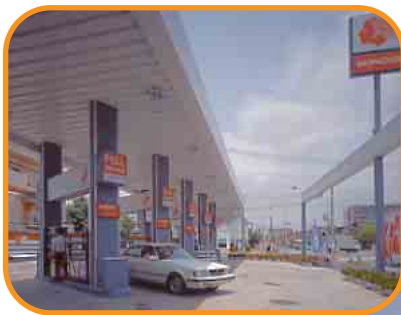
A sinanen service station
