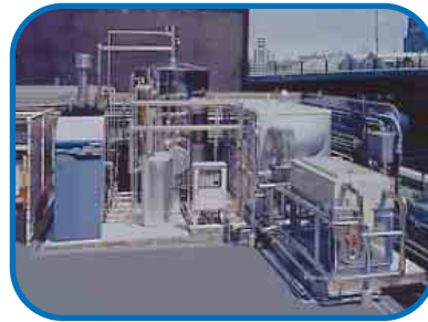
Sinanen’s micro gas-turbine co-generation system ensures more efficient use energy and environment friendly.
