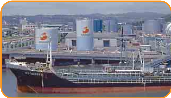
Sinanen's oil storage facilities located in shiogama, miyagi prefecture.
