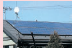
Photovoltaic Power System
