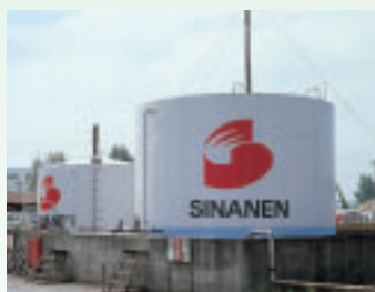
Kerosene Tank Sagamihara Sales Office
