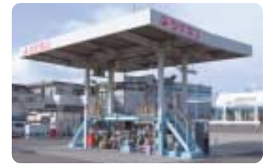
Ougimachi Kerosene Depot, Miyagi Prefecture
