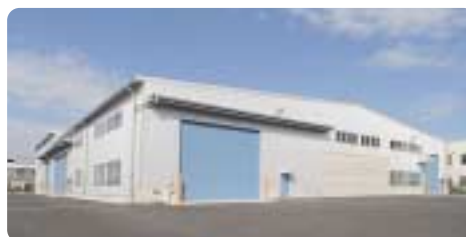
Biomass Fuel Production Plant (Chiba Recycling Center)
